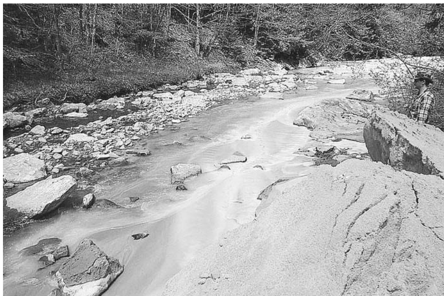
PLATE 1. Limestone sand treatment of First Fork to Shavers Fork in the Cheat River watershed, West Virginia, USA. Photo credit: Pete Lamothe.
